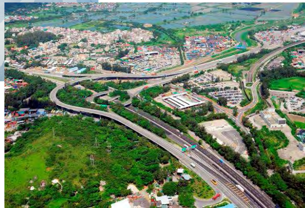
Improvement Works to San Tin Interchange
