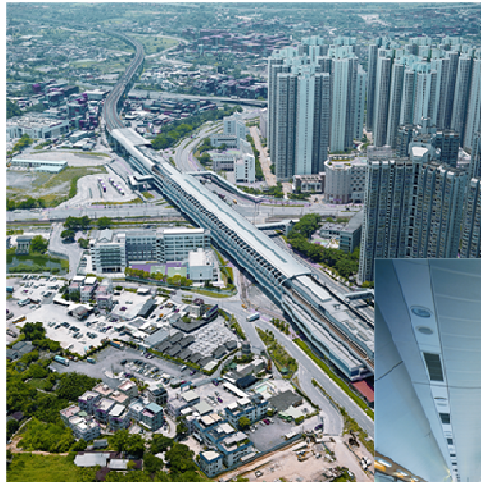
West Rail Kam Tin to Tin Shui Wai Section Viaduct
