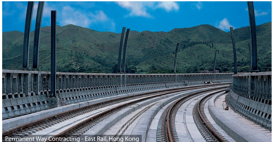
Permanent Way Contracting - East Rail, Hong Kong
